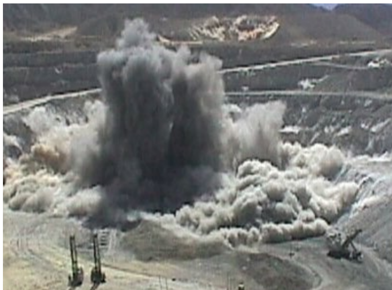
Figure 4 Failure to Contain Explosion Energy
